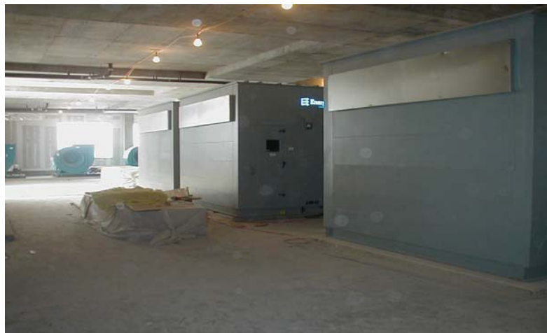
INOVA Photo 1: “Mechanical Penthouse,” August 12, 2003
