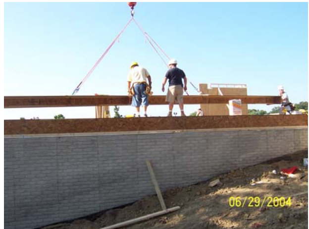
Figure 9: A first floor panel being installed.
