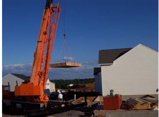
Figure 7: Panel being picked with a crane.
