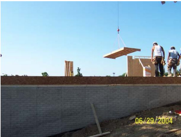
Figure 8: A first floor panels being swung into place.
