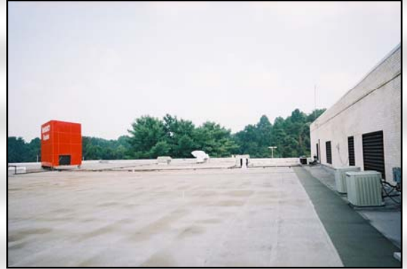
First Floor Roof
