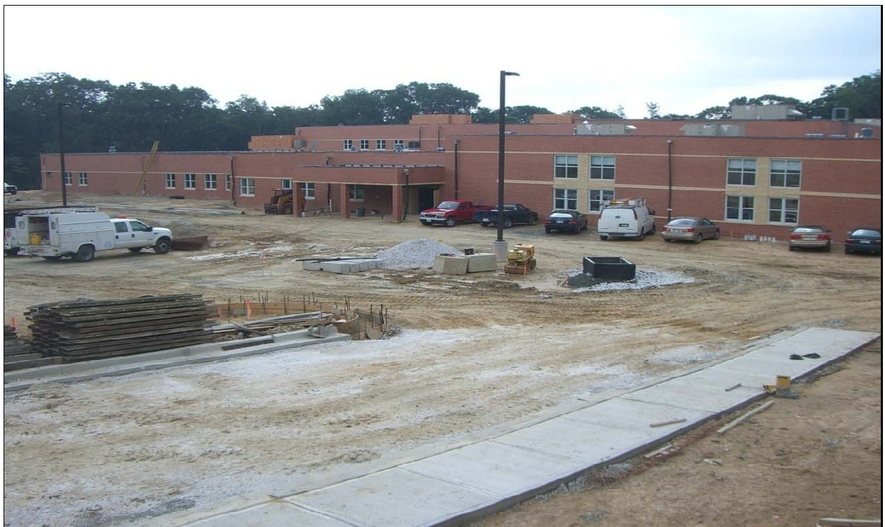
Building Exterior at Main Entrance
