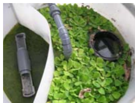
Figure 24: Clarifying Tank Located at Penn State’s Center for Sustainability
