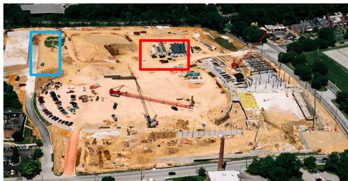
Figure 16 - Site Picture during Excavation
