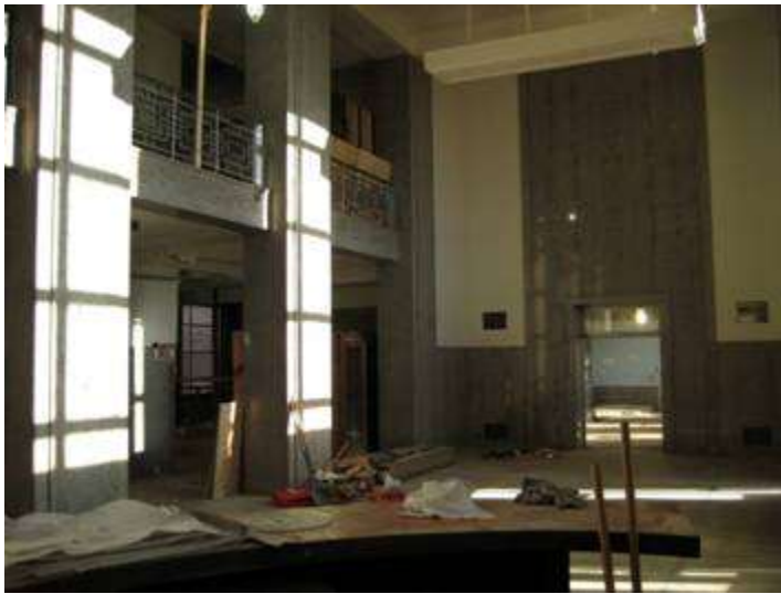
Before renovation, with surfaces being stripped
