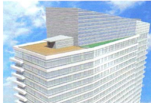
Figure 1. A 10,000 ft 2 green roof highlights the environmental designs of The Helena.
