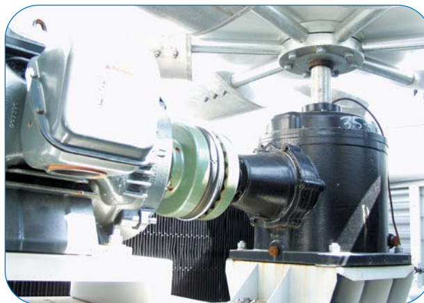
Gear Drive System, Close-Coupled Motor
