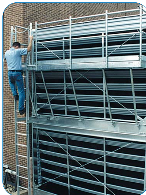
External platform at louver face
