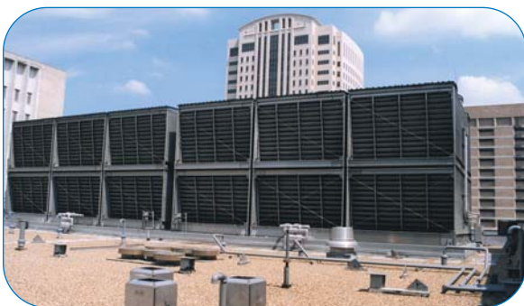
Basinless Series 3000 Cooling Tower on a concrete basin
