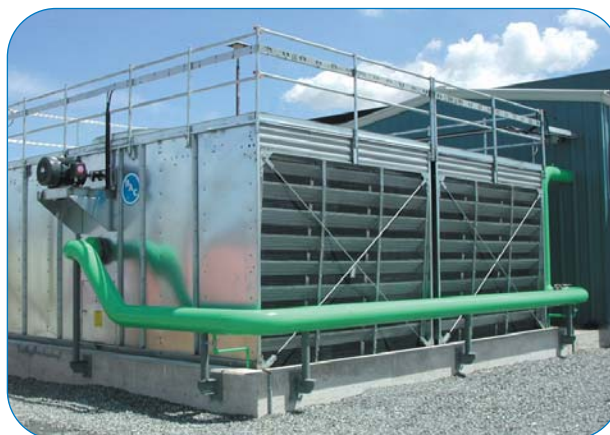
Gear Drive System, Externally Mounted Motor
