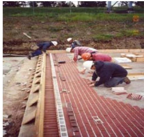
Figure 1: Laying the thin bricks
