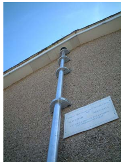
Figure 3 - Correctly assembled & installed mast mounting brackets
