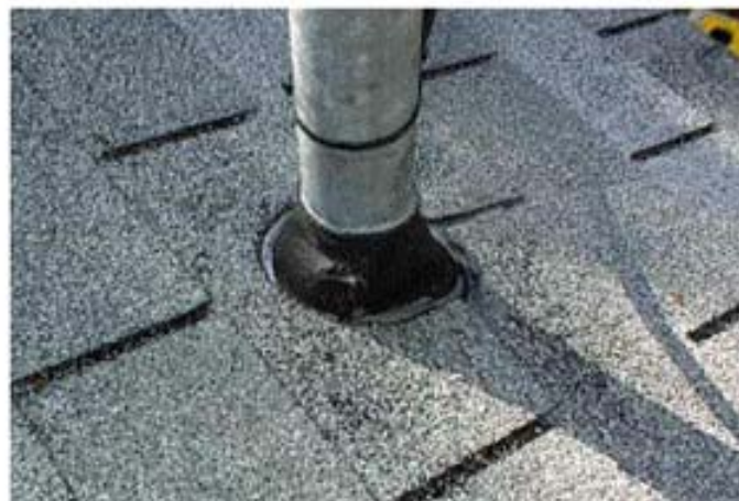
Figure 5 - Typical installation of rubber roof gland seal.
