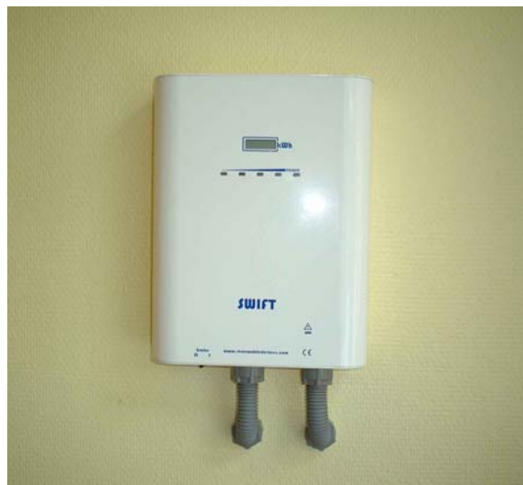
Figure 7 - Installed SWIFT™ Electronic Control System
