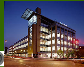
PNC Firstside Center
