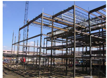
Figure 2 - Steel erection underway
