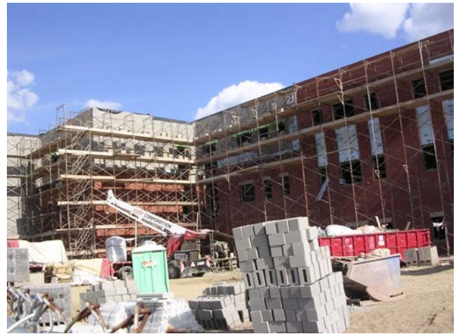
Figure 1 - Mason scaffolding around building footprint.
