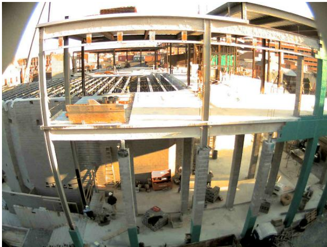
Figure 66: North-facing Construction Photograph Showing Original Joists Above Recital Hall
