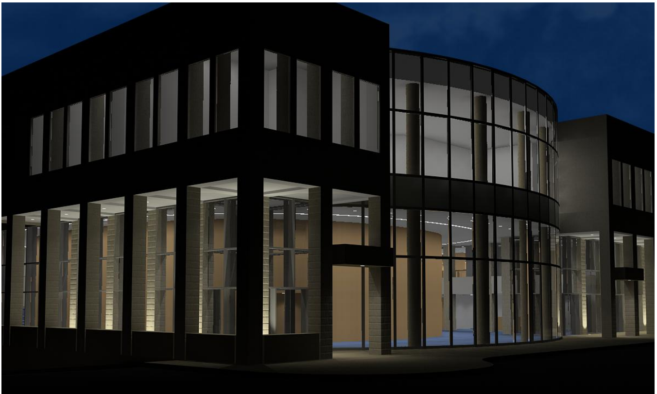
Figure 6: Building Entrance, Corner Perspective View
