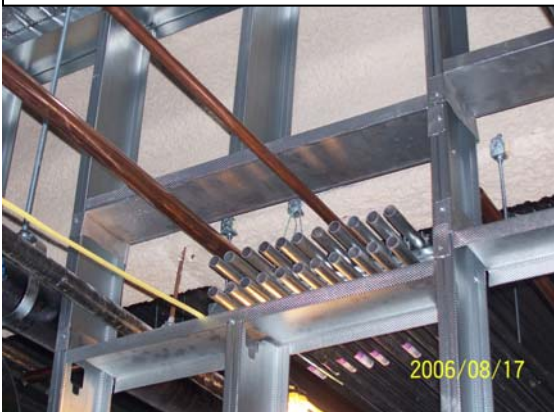
Figure 10 – 5 th Floor MEP Rough-in
