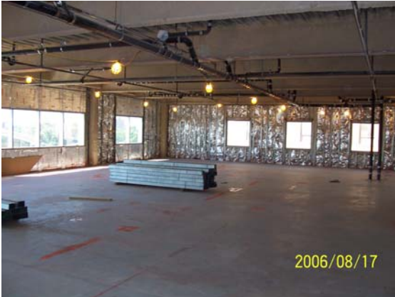
Figure 9 – 6 th Floor Shell Space
