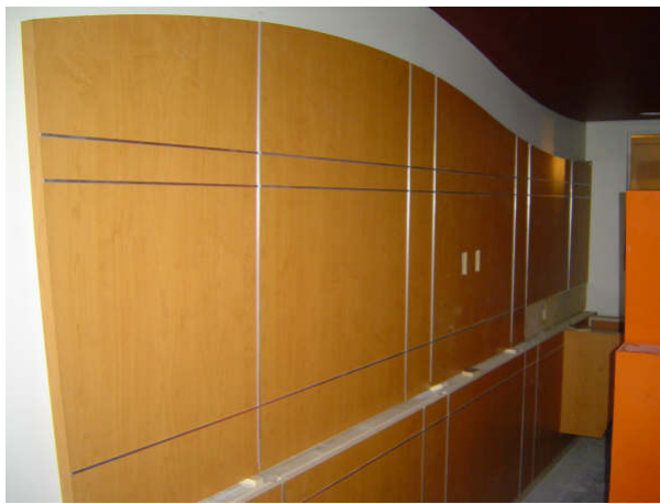
Figure 12 – 5 th Floor Patient Room Finishes
