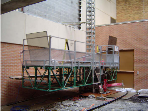
Figure 6 - Self Climbing Scaffold
