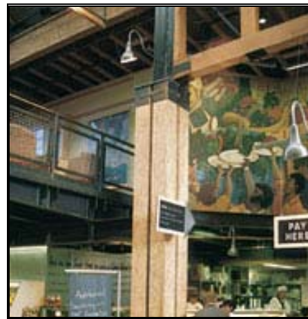
Figure 32: Engineered Wood Column Sample 4
