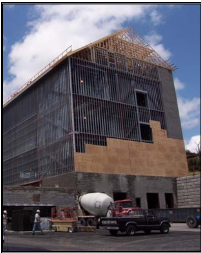
Figure 2: Light gauge steel framing with plywood sheathing 1
