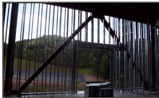
Figure 8: Frame with tube chevron bracing 1
