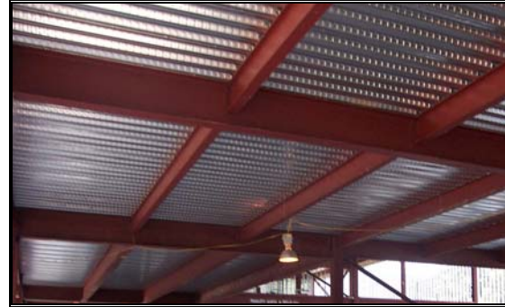
Figure 5: Composite slab as placed during construction 1
