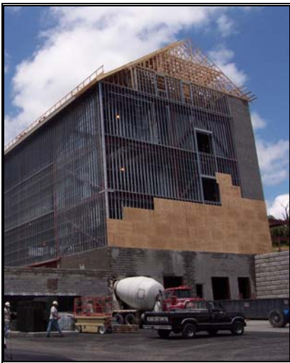
Figure 2: Light gauge steel framing with plywood sheathing 1
