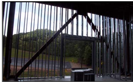
Figure 8: Frame with tube chevron bracing 1
