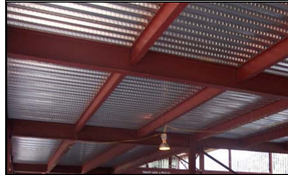
Figure 5: Composite slab as placed during construction 1
