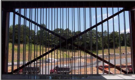
Figure 7: Frame with double angle cross-bracing 1
