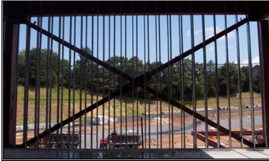
Frame with double angle cross-bracing 1
