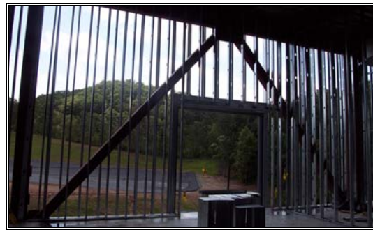
Frame with tube chevron bracing 1
