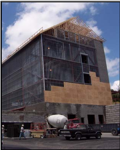
Light gauge steel framing with plywood sheathing 1
