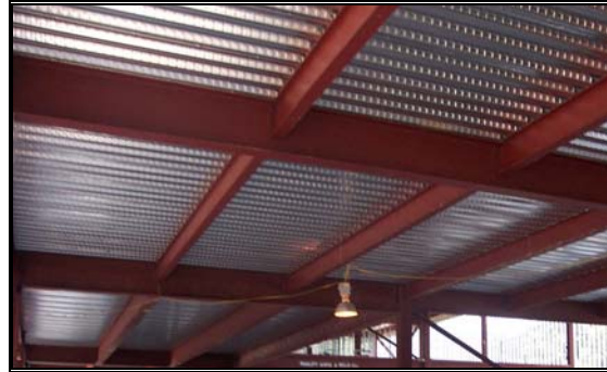
Composite slab as placed during construction 1
