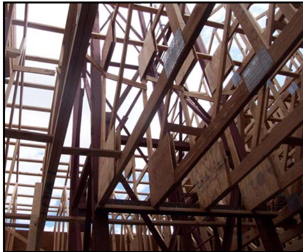
Roof trusses of 2x4 No.2 Southern Pine spaced at 2' OC. 1
