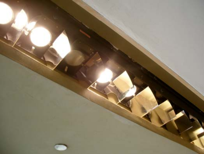
Replace incandescent perimeter lighting
