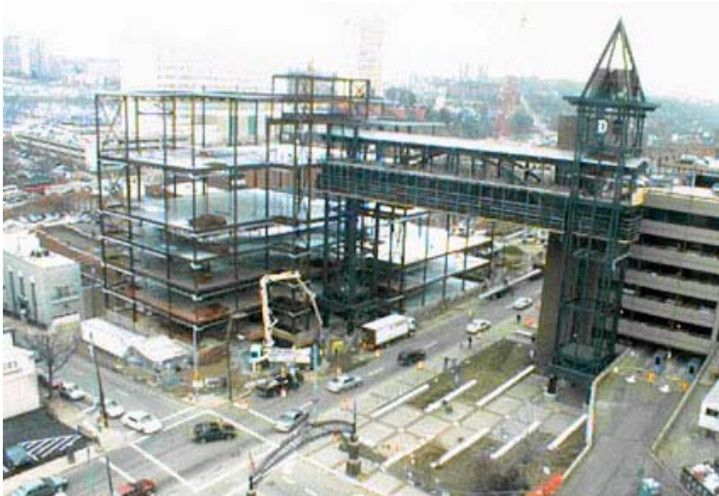
Construction as of November 2006
