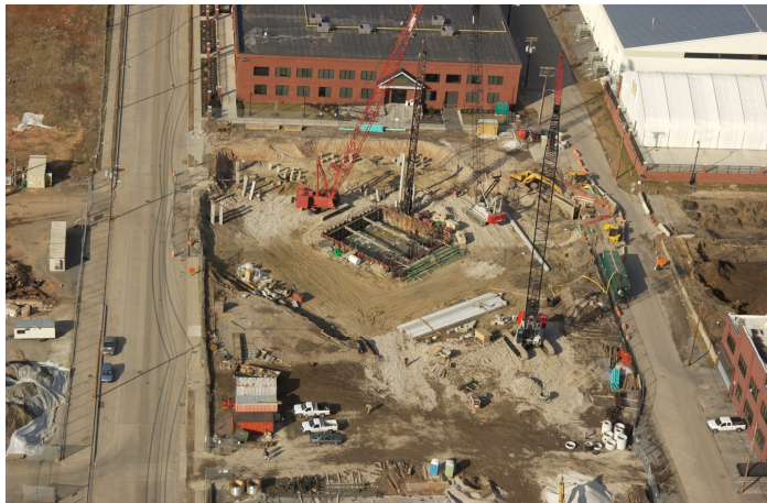
Fig 4– Aerial view of existing site conditions
