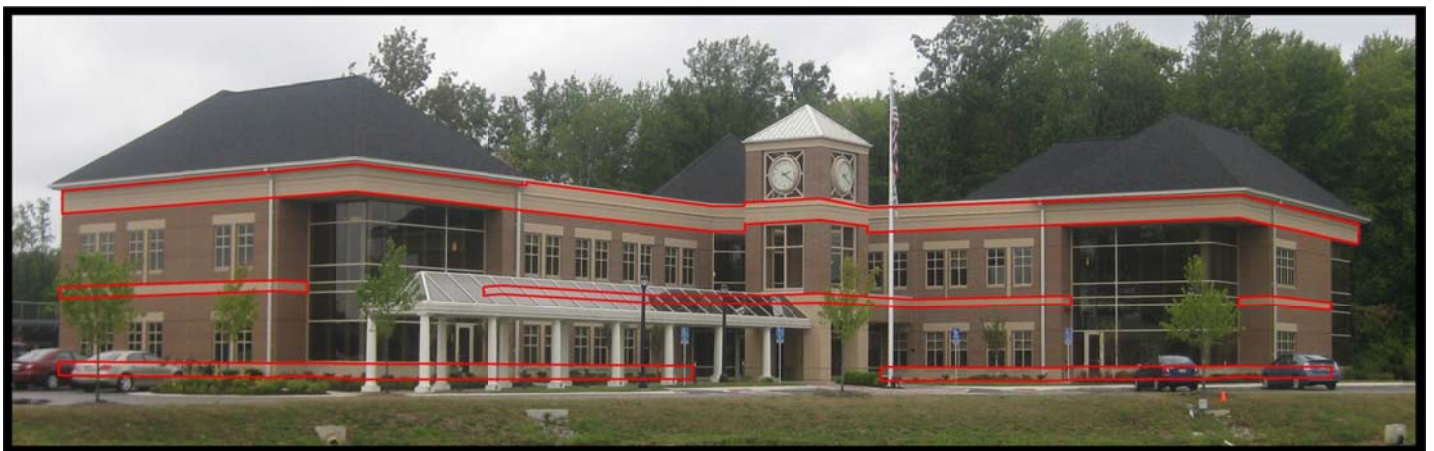
Lines of Horizontal Tan Brick on Building Façade
