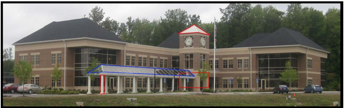
Entrance Structure Architectural Problem Areas
