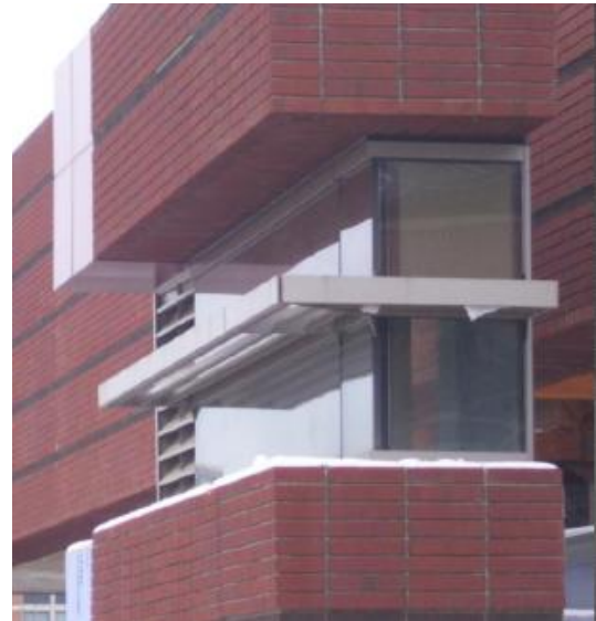
Figure 2: Mockup of building enclosure, including pre-cast panels
