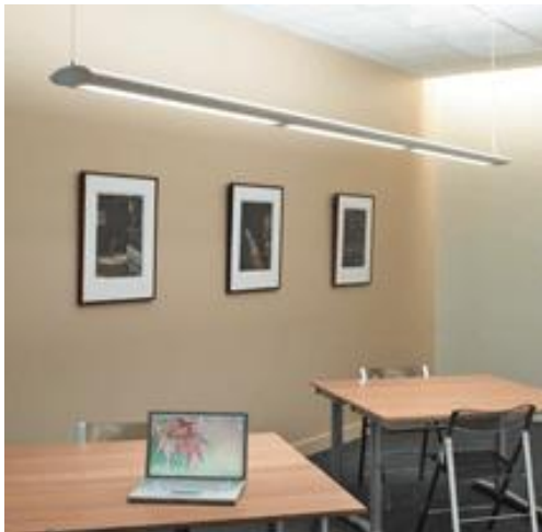
Figure 12: Indirect-direct lighting application
