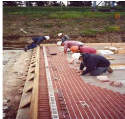
Figure 1: Laying the thin bricks
