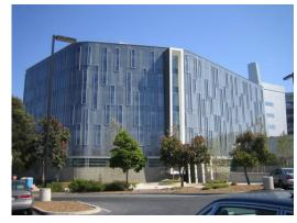
aluminum cladding for the mullions, and various types of clear vision glass panels for the windows spanning vertically and horizontally are used.
