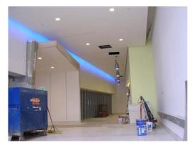
Suspended fluorescent T8 fixtures are used for open office areas along with recessed strip lights in private offices and some corridors. As can be seen, because of the variety of spaces for this building, the lighting was designed to coordinate with each separate space while also integrating each space into the next with similar lamps, feels, and ambience.
