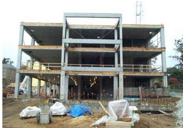
Typical elevation during the construction of the KINSC
