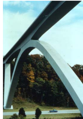
Figure 11: Post-tensioned bridge span
