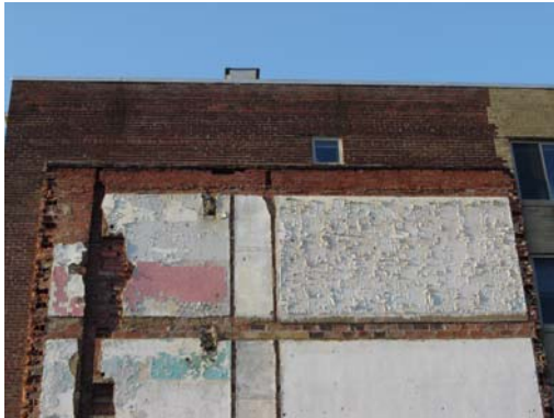
Existing Apartment Wall
