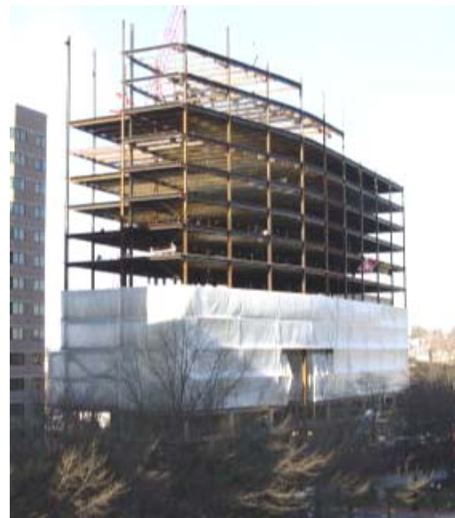
Figure 9 -Steel framing during construction. (Photo courtesy of Gilbane)
