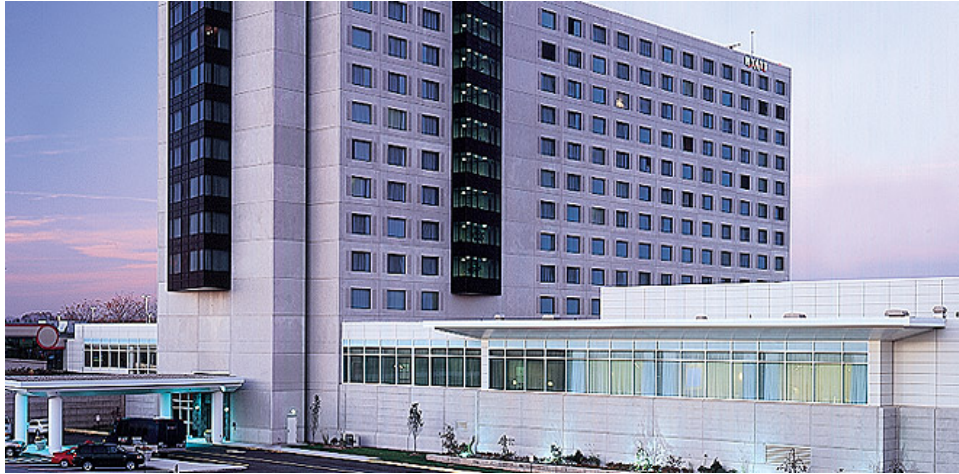
Figure 1. – Exterior of Building Tower (left) and Conference Center (right)
