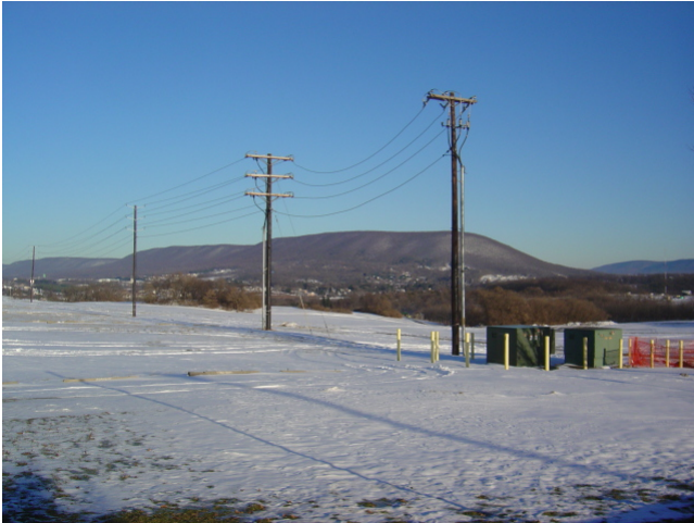
Overhead High-Voltage Power Lines on Site
