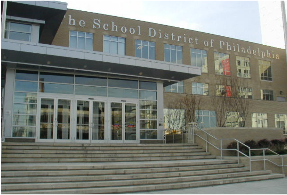
Figure 1.1D. Broad Street Entrance.
