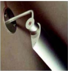
End mounting brackets may be modified to suit unique conditions.
