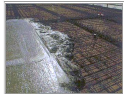
First Floor Slab
