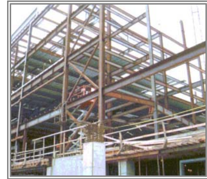
Lateral Cross-Bracing
