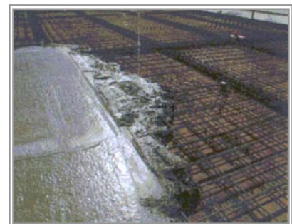
First Floor Slab
