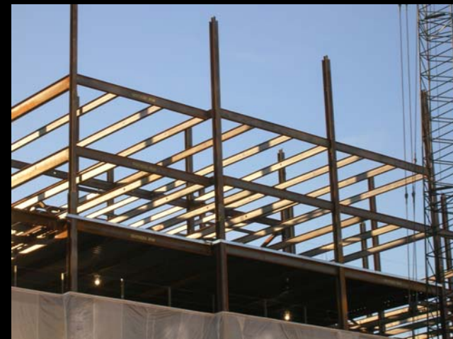
Composite Beam Floor System
