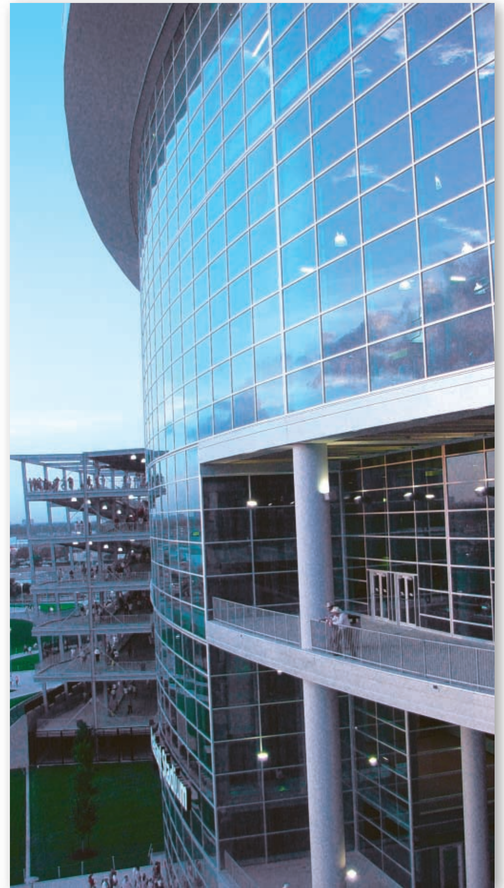
Houston Texans Reliant Stadium All upper areas: Pilkington 1/4" tempered Blue Green
