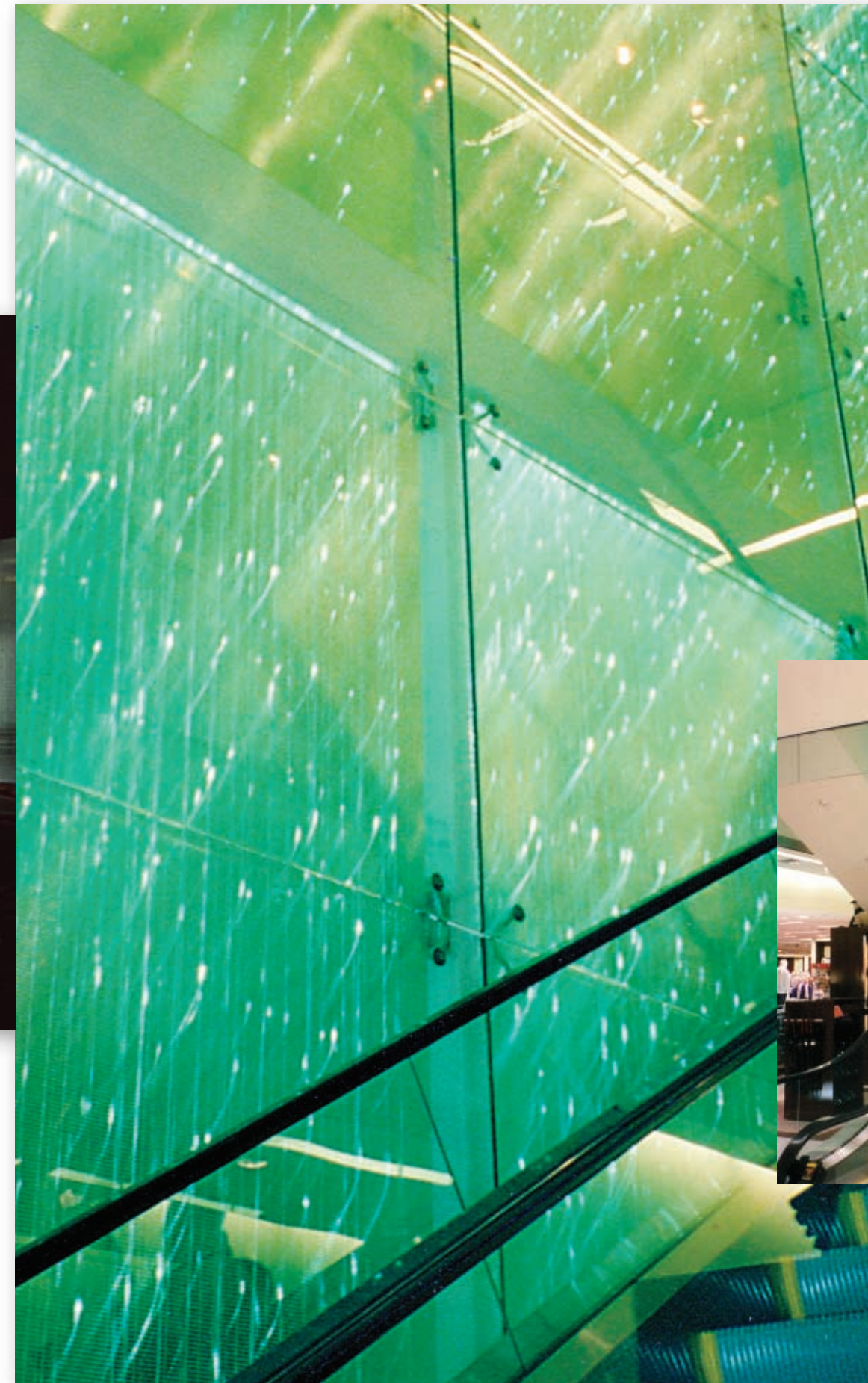
Bloomingdale's - Orlando, Florida Laminated patterned glass set in engineered Point Supported Wall System, with diode back-lighting
