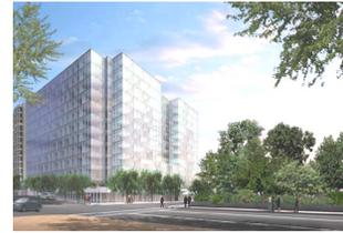
The building is located in downtown Washington, DC. This is an urban setting, which is reflected in several factors in lateral load determination. Its primary use is for standard office tenants, and just meets DC height restrictions at 12 stories and 128 feet. Gravity loads are resisted by a two-way flat slab with drop panels poured around the majority of columns. The slab contains post-tensioned tendons for additional stiffness and an enhanced stress profile.
