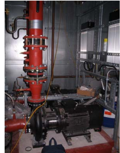
Fig 3.8 Central Boiler Plant
