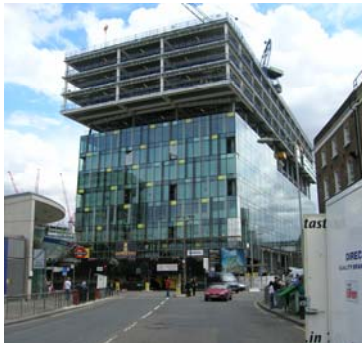
Figure 3.1 Palestra under Construction
