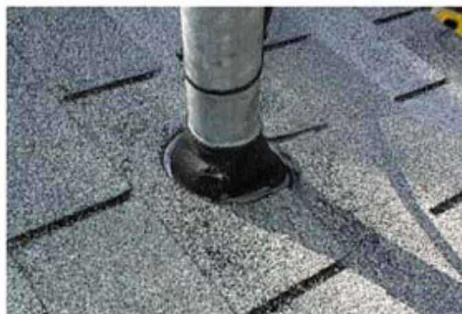
Figure 5 - Typical installation of rubber roof gland seal.
