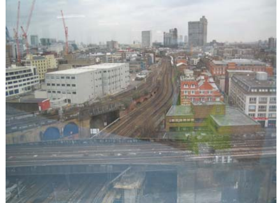
Figure 7.5 View of High Traffic Areas from 7 th Floor
