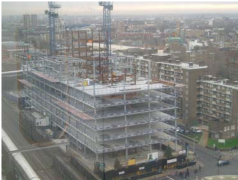
Fig 3.9 Steel Framework of Palestra
