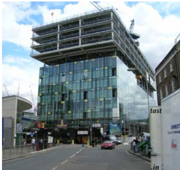
Figure 3.1 Palestra under Construction
