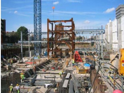
Figure 3.5 Steel Erection on Palestra Site
