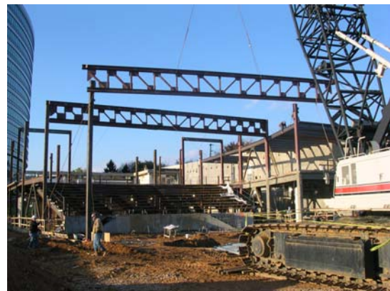
Figure 10. Placement of Steel Trusses
