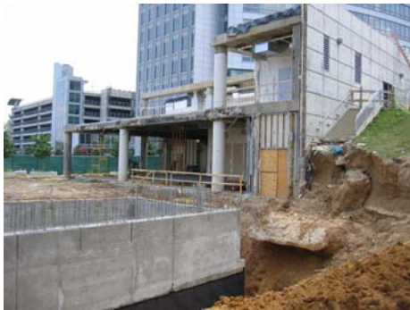
Figure 3. Base Building Demolition
