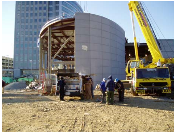
Figure 7. Installation of Pre-cast Panels
