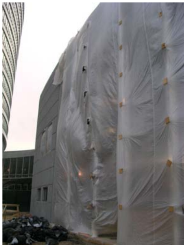
Figure 8. Future Curtain Wall Location
