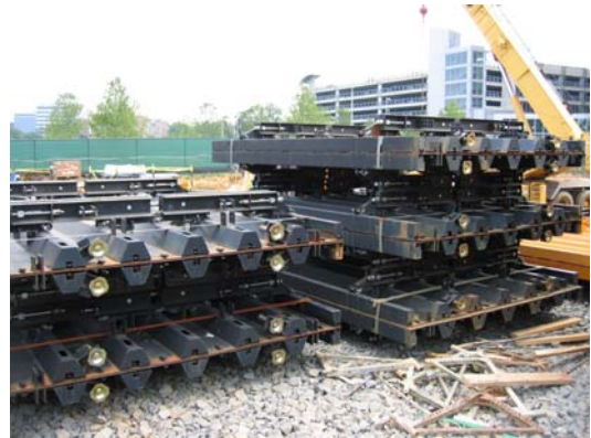
Figure 5. Ulma Forms in Staging Area
