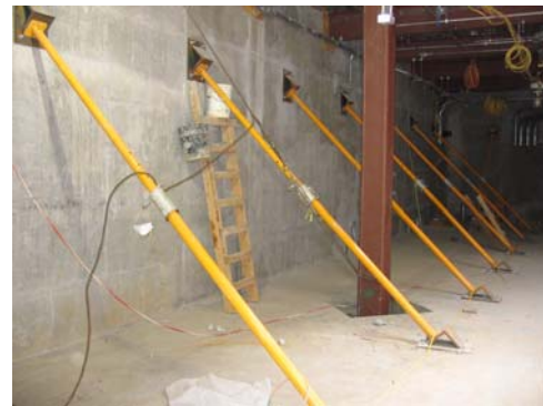
Figure 13. Ulma Raker Support
