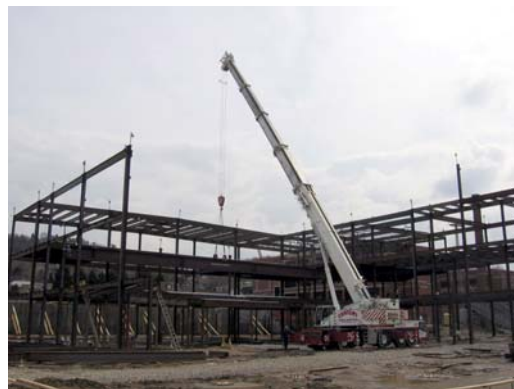
Figure 4 - Erection of Plate Girder
