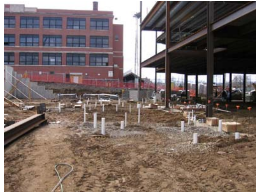
Figure 2 - Basement Slab on Grade
