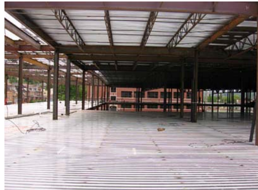
Figure 7 – 2 nd Floor Decking installed ready for slab pour
