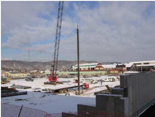
Figure 1 - Erection of 1 st Column
