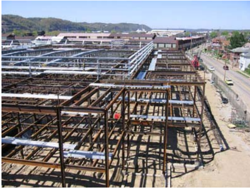
Figure 5 - Structural Steel Complete, Metal Deck Beginning
