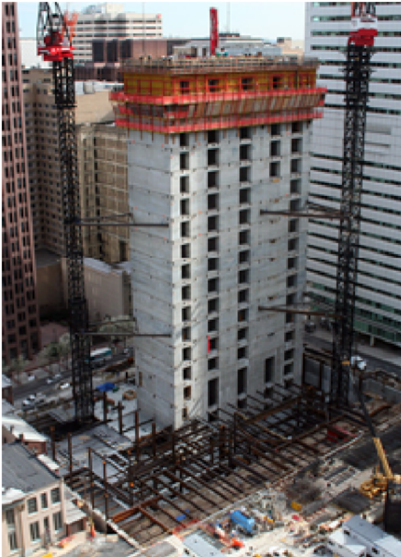
CONCRETE CORE CONSTRUCTED FIRST, STEEL ERECTION FOLLOWS
