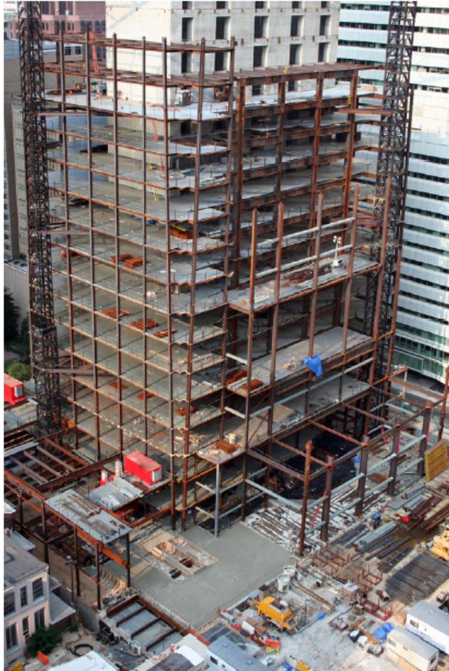
COMPOSITE SLABS DECREASE FLOOR SYSTEM DEPTH
