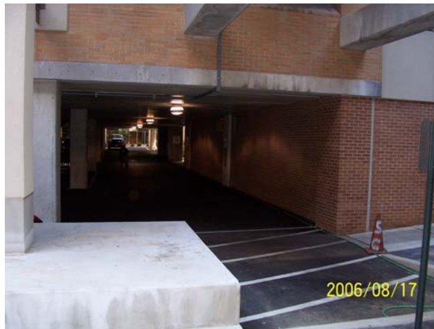
Figure 14 - Access to Elevator Site
