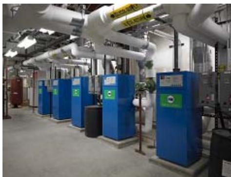
Figure XXIV – Boiler Systems located in Mechanical Penthouse
