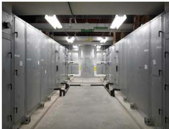
Figure XXI –AHU-1 and AHU-2 Located in Mechanical Penthouse
