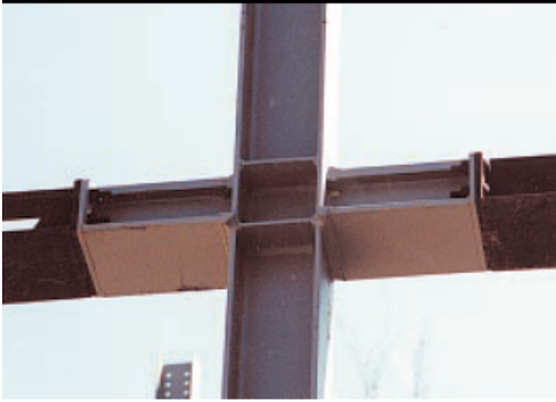
Figure 6 Typical "Gooseneck" Connection
