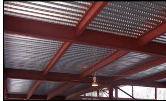
Figure 5: Composite slab as placed during construction 1
